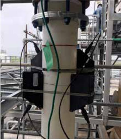
*Redundant clamp-on flow sensor installations on Kynar spool*
