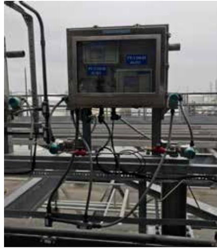
*Redundant FUG1010 meters housed in a stainless enclosure along with Siemens pressure and temperature instruments*
