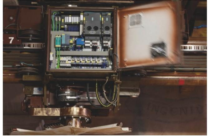
Control box installed on gondola including fail-safe SIMATIC PLC and fail-safe frequency converters.
