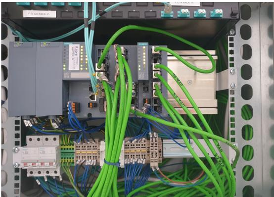
SCALANCE XM416-4C: the core of the production backbone that provides high availability and redundancy to the plant network.
