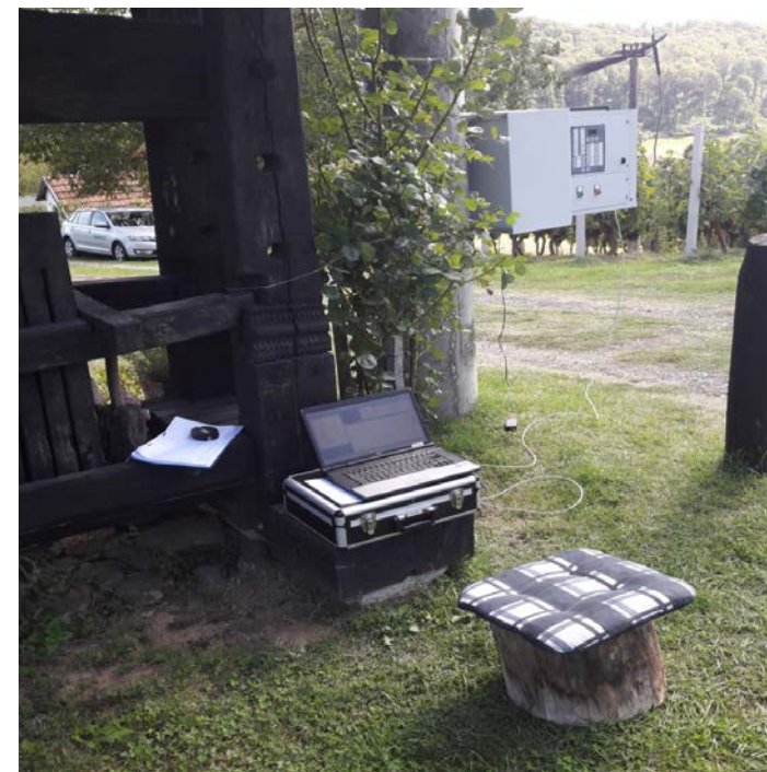
Signal testing and energizing of 3AD recloser 1 (Master)
