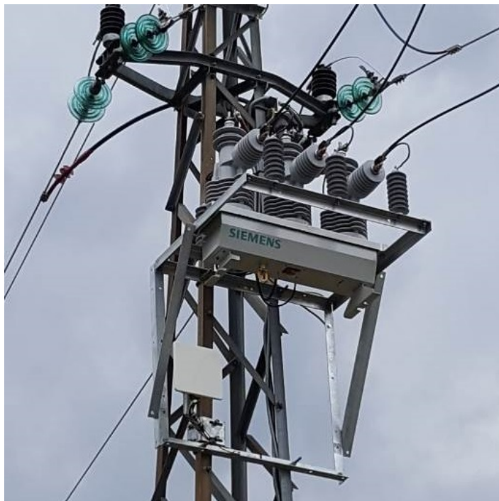
3AD Recloser and Communication antena
