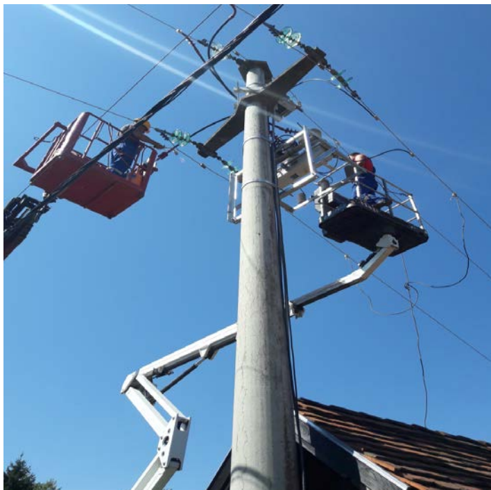
Instalation period of 3AD recloser RC2
