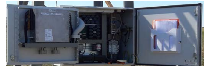
Factory test of complete solution, Zagreb
