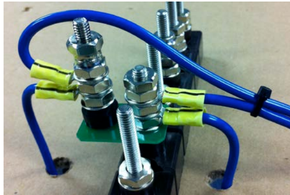
Figure 2-2 Installed Current Sensor Adapter
