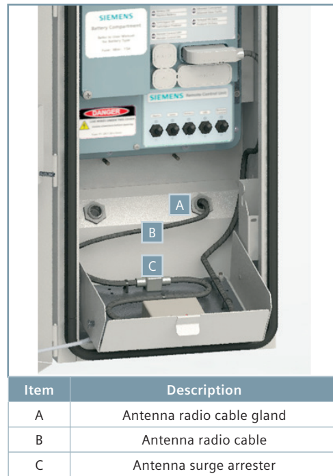
Figure 33: Antenna cable connection
