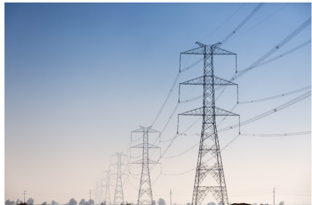
Figure 2 - Egypt Megaproject Substations
