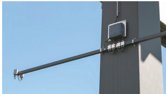
The SCALANCE W786 Access Points are installed on the supports of the railway and communicate via two antennas on outriggers with the trains on the two tracks.
