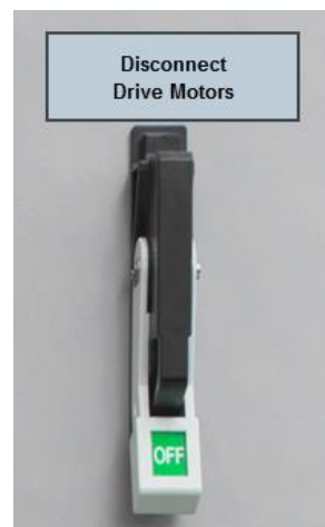
Supply circuit disconnecting means for drive motors
