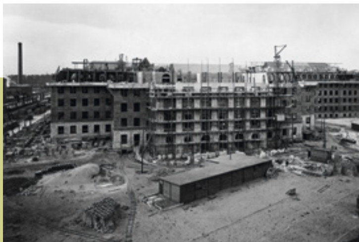
At the heart of Siemensstadt – construction of the Siemens-Schuckertwerke administration building at the intersection of Nonnendammallee and Rohrdamm, February to December 1913
