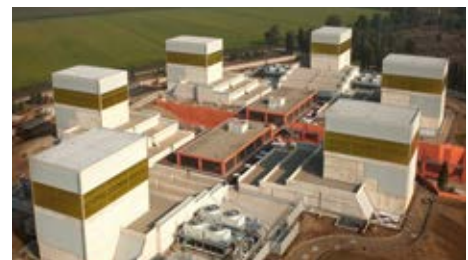
Das Eni Green Data Center in Ferrera Erbognone
