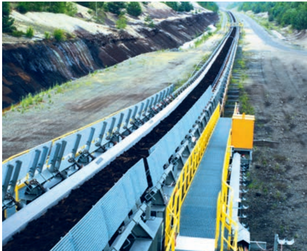
Overland conveyor at an open-pit mine, Reichwalde, Germany
