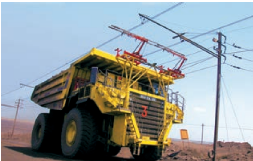
Using trolley-assist from Siemens, fuel consumption and thus CO 2 emissions can be cut significantly
