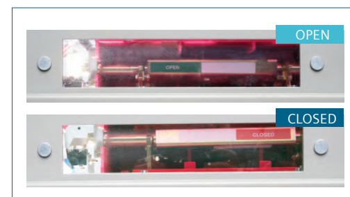
Viewing window for isolating switch position
