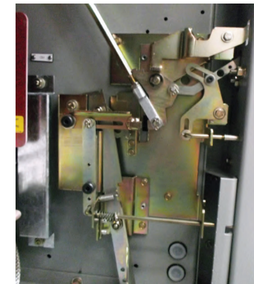
Isolating switch operating mechanism
