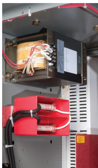
Control power transformer mounted in the cell
