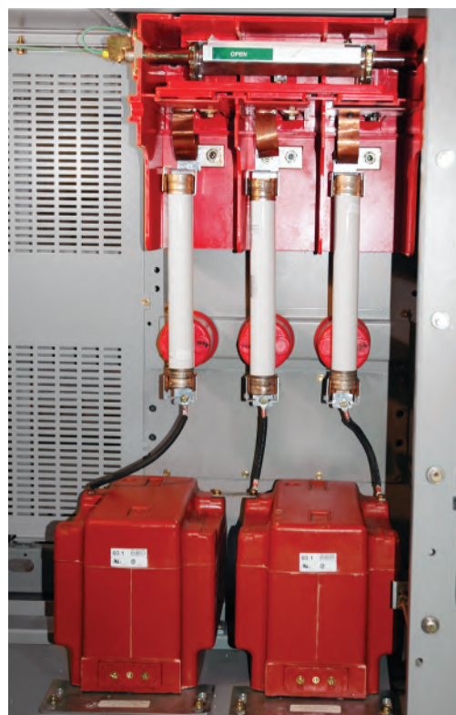
Voltage transformer for incoming line or main bus VTs
