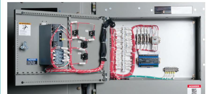
Inside view of low-voltage/control compartment
