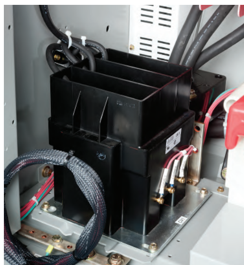
Voltage transformer arrangement in the feeder cell
