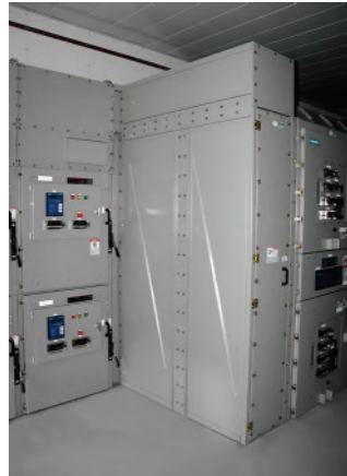
PRC integrated into transition between GM-SG-AR and SIMOVAC-AR
