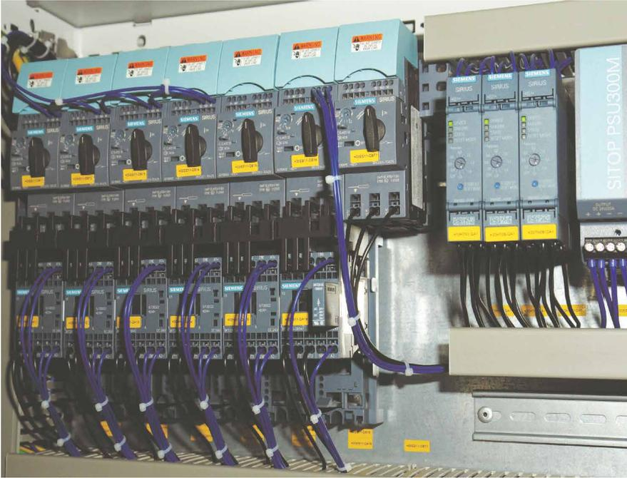
The Siemens 3RV29 infeed system is much less labor intensive.
