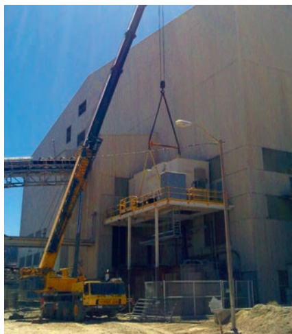
Installation of new container (E-House) outside of the grinding building
