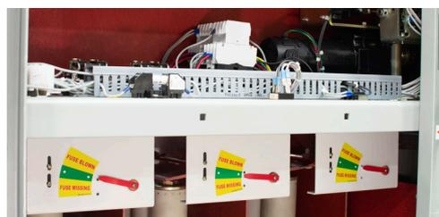
Blown fuse window with indication flags and motor-operated switch, shown with main door open
