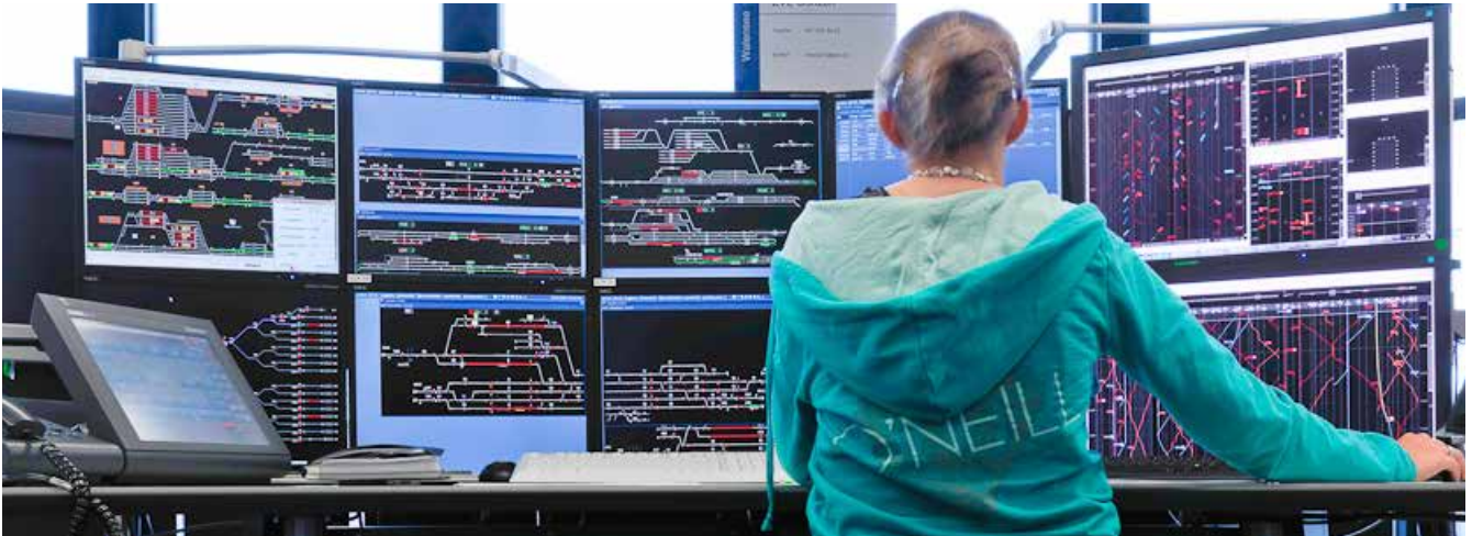
Iltis N operation centre
