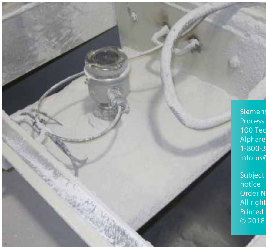
SITRANS LR560's highly durable polyetheramide lens antenna (left) can tolerate significant buildup, such as kiln dust
