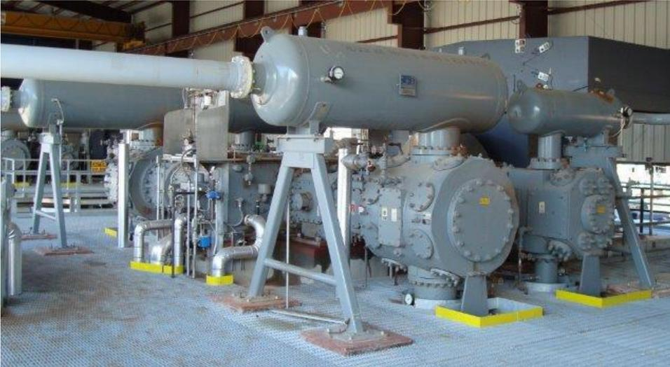
**Above:** Typical Dresser-Rand® HHE-VL reciprocating compressor installation utilizing an engine-type synchronous motor similar to the configuration of the three units that will be installed at the new steam methane reformer (SMR) in Texas.
