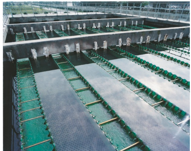
With LTE, remote wells in rural areas, silos, or sewage treatment plants can also be continuously monitored.
