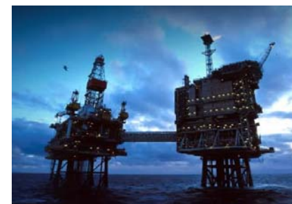
Main application: Offshore production platforms
