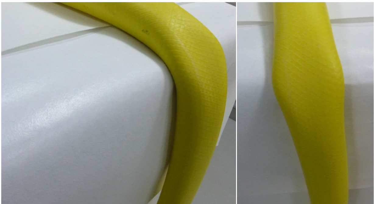
Figure 20-Incorrect routing (hose deformed over “sharp” edge- Gorilla 1.5” Hose)
