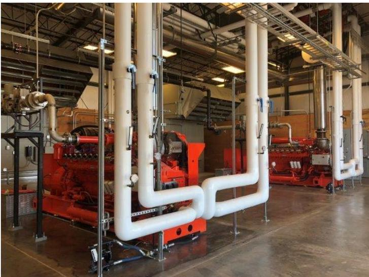
**Above: Siemens SGE-56HM engine provides customers like SISW with a high-performing low-operating-cost solution.**
