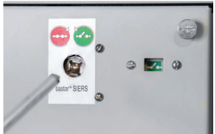
Figure 13: Inserting \frac{3}{8} " drive extension into SIERS drive socket
