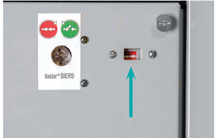
Figure 15: SIERS system position indicator in CONNECTED position
