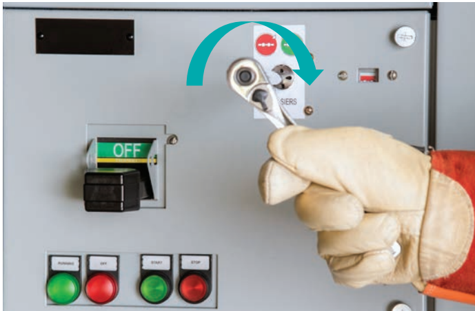
Figure 14: Rotate tool clockwise to extend stabs and place the SIERS' system in the CONNECTED position
