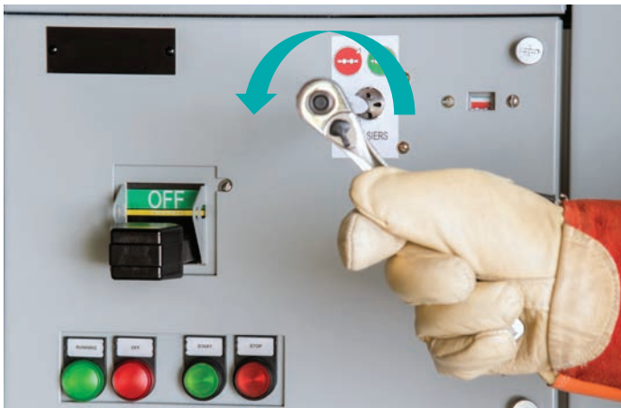
Figure 16: Rotate tool counter-clockwise to retract stabs and place the SIERS' system in the DISCONNECTED position
