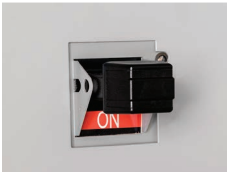
Figure 10: Operating handle position: ON
