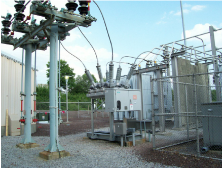
Installation of a Siemens 69kV SPS2 circuit breaker
