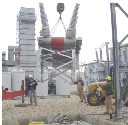
Installation of a Siemens 145kV SPS2 circuit breaker
