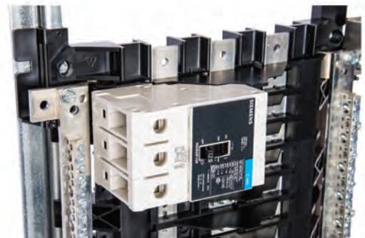
Example of Back-fed NGB Main breaker installed
