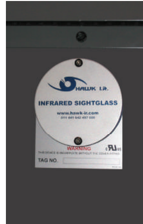
Infrared viewing ports
