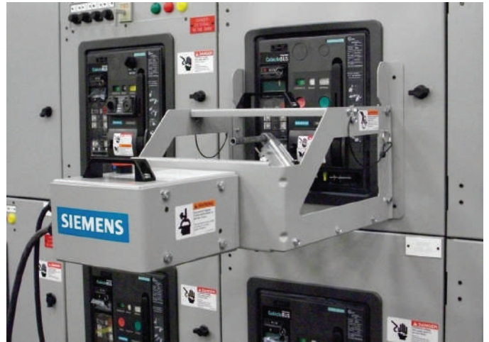
Remote Racking Device
