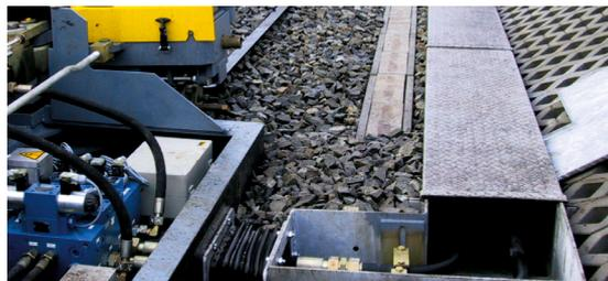
Active water protection with piping installed in oil-tight ducts
