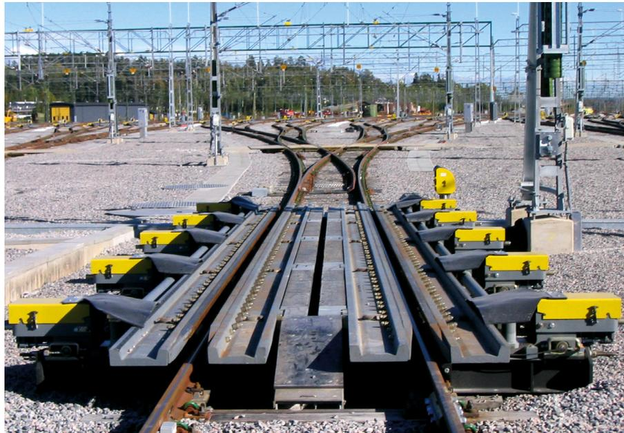
The process of joining cars in the exact position for coupling with due regard to their load is also a major requirement on classification tracks with respect to target-shooting. In order to meet this requirement and use these benefits for customers, retarders and the Trackguard Cargo MSR32 control system have been combined to form a highly efficient system for many years now.
