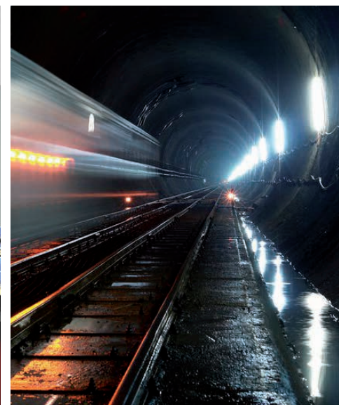
The tunnel control system will be ready for operation from the summer of 2015.
