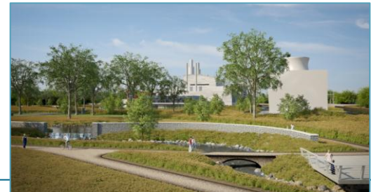
Holland Energy Park, Michigan 2 Siemens SGT-800, steam turbine and generator
