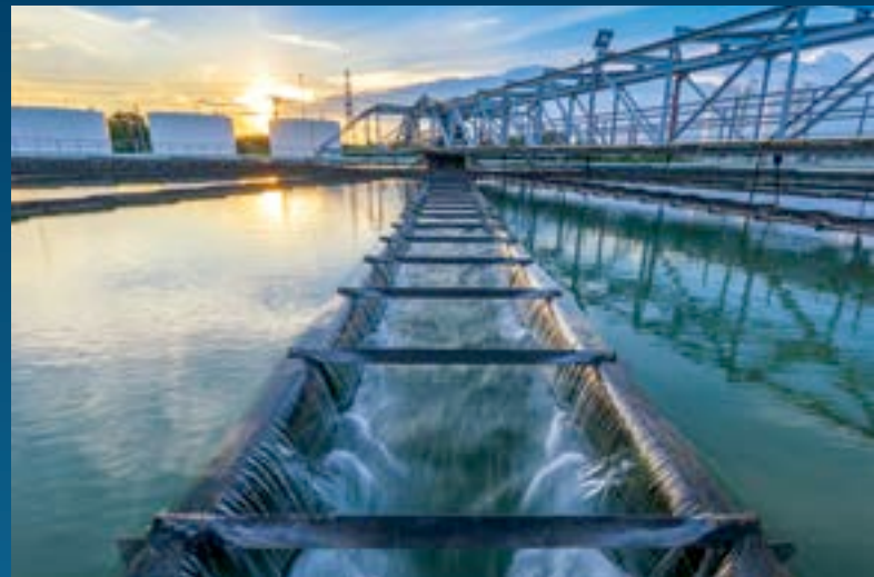
Wastewater treatment plant
