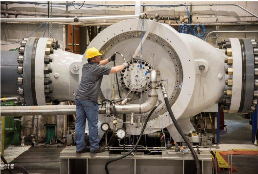
RFBB36 Pipeline Verdichter.
