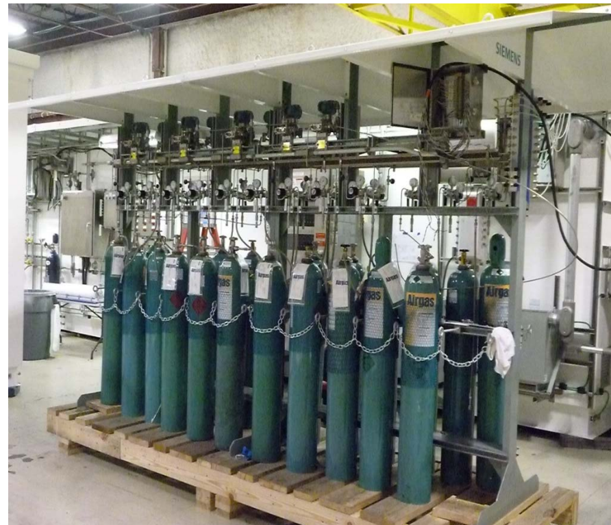
Open Air Cabinet for Flare MassSpec Calibration/Validation
