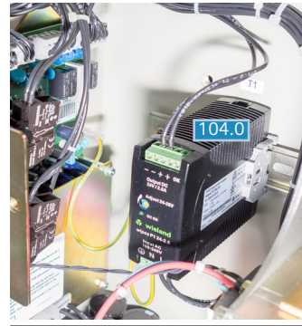
Figure 23: Power supply replacement
