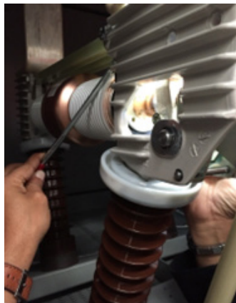
Figure 18b: How to view contact erosion indicator between poles
