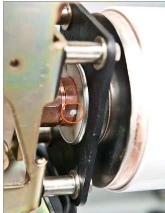
Figure 18a: Contact-erosion check mark dot circled in orange (shown with circuit breaker CLOSED)
