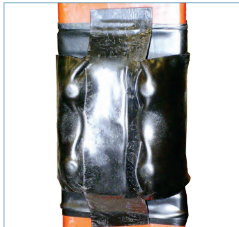
Figure 26: Typical installation of insulating boots
