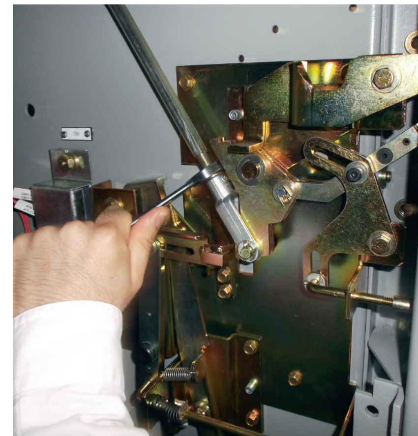
Figure 72: Isolating switch - connecting rod adjustment for correct DSI switch operation
