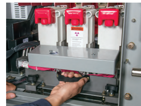
Figure 42: Installing type 12SVC400 (400 A) contactor
