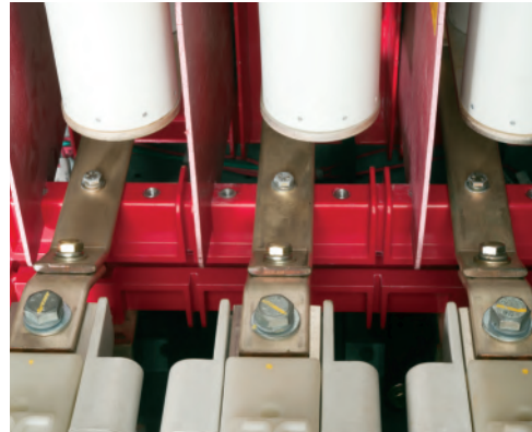
Figure 44: Installing type 12SVC400 (400 A) contactor - high-voltage connections for fixed-mount design
