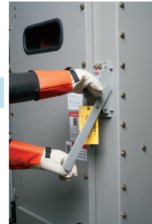
Figure 60: Operation of load-interrupter switch
