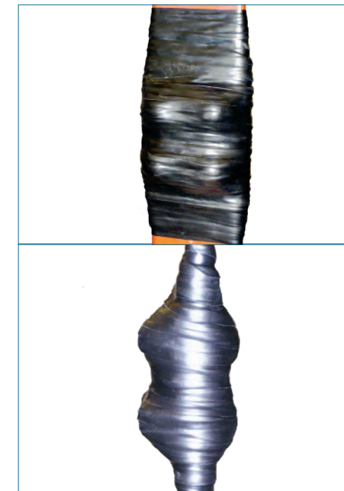
Figure 29: Final insulation
