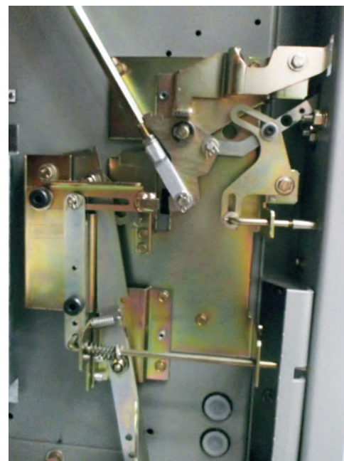
Figure 50: Isolating switch operating mechanism
