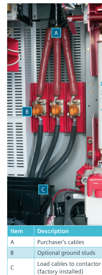
Figure 31: Typical outgoing connections
