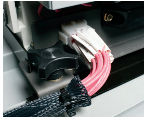
Figure 46: Installing type 12SVC400 (400 A) contactor - connecting compartment umbilical cord
