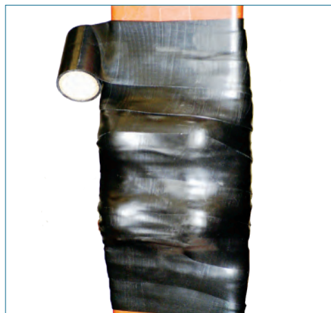
Figure 28: Insulation with half-lapped tape
