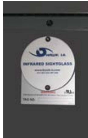
Infrared viewing ports
