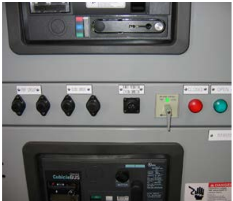
Control port on WL Switchgear
