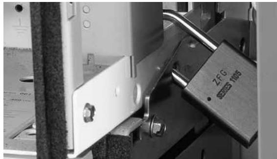
Figure 62: Padlocking in "test" position
