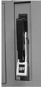
Figure 59: Operating handle in "OFF" position
