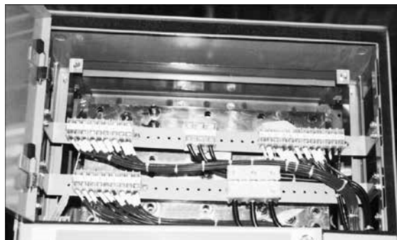
Figure 46: Type “C” wiring terminal
