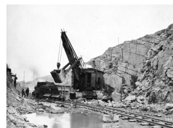
Excavation, rock removal, 1927
