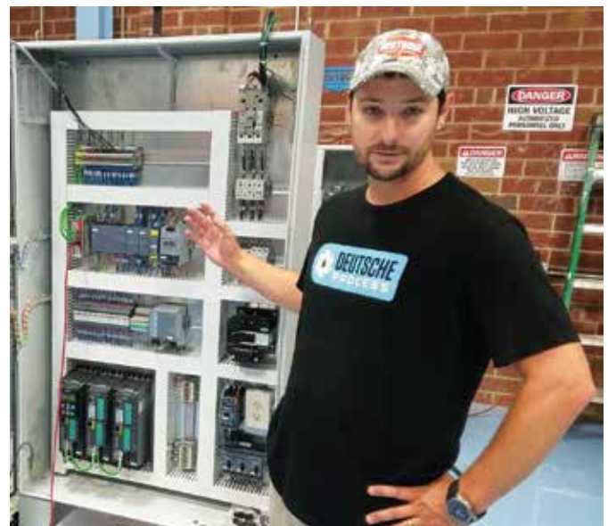
Cameron Cane, Deutsche Beverage explains Siemens products within the Deutsche Beverage-built control cabinet.
