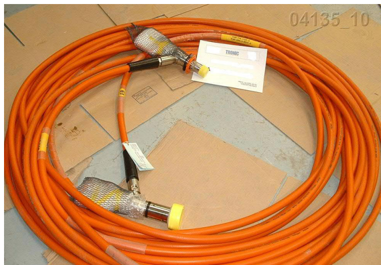
Figure 4 Image to show Electrical Flying Lead.
