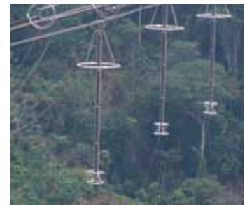
550 kV line in Colombia NGLA solution realized with 3EL2
