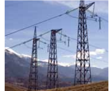
400 kV line in Bulgaria NGLA solution realized with 3EL2
