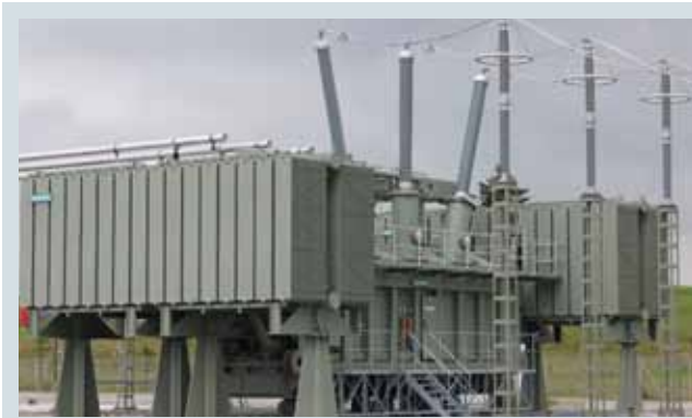
Substation Bidingen 400 kV
