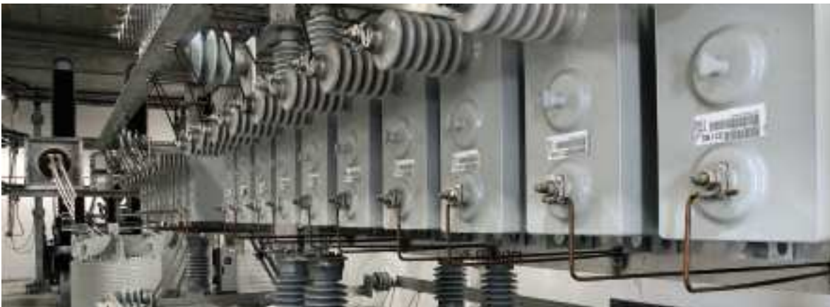
Key components of a PTD power-factor correction system that is stabilizing the electricity transmission network in southern Denmark.
