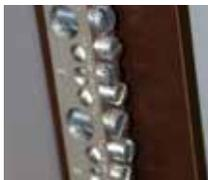
Outboard neutral and groundbars allow for all connections to be located away from the breaker connections, making for a neat, clean installation.
