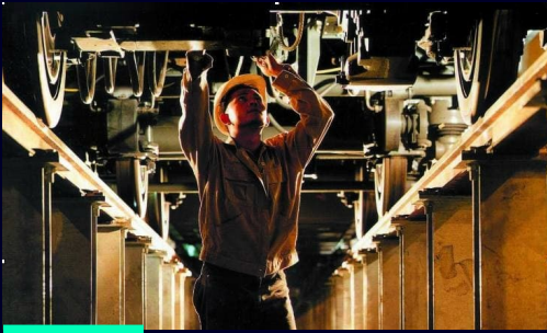
Customer Services Servicing of Traction control converter
