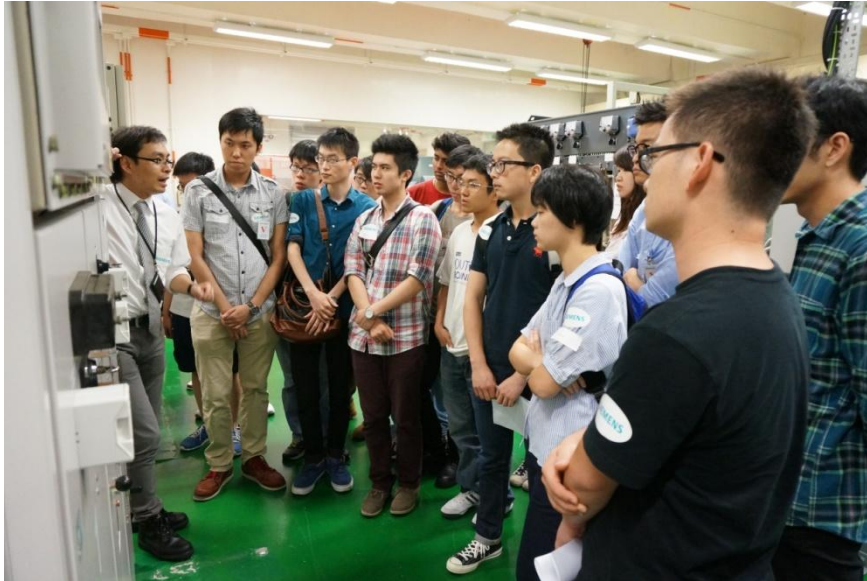
Experienced engineers from Siemens introduced the company's switchgears which are currently operated in our customer's power substations.
