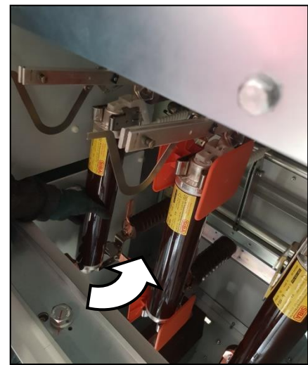
Fig. 422: HV HRC fuse-link inserted on the opposite side of striker area
