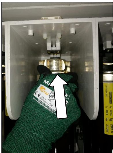
Fig. 255: Opening the fuse-link bracket in the striker area (operating side of contactor truck)
