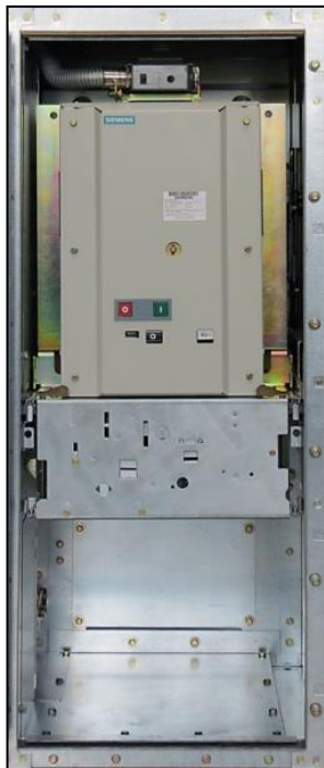
Fig. 113: Circuit-breaker panel with high-voltage door open (type 3AE5 as an example)
