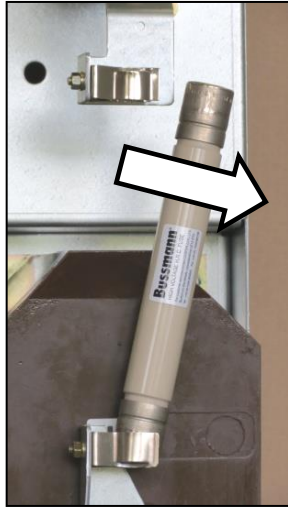
Fig. 171: Pulling off the fuse-link
