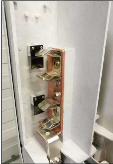
Fig. 249: HV HRC fuse-link removed in the striker area
