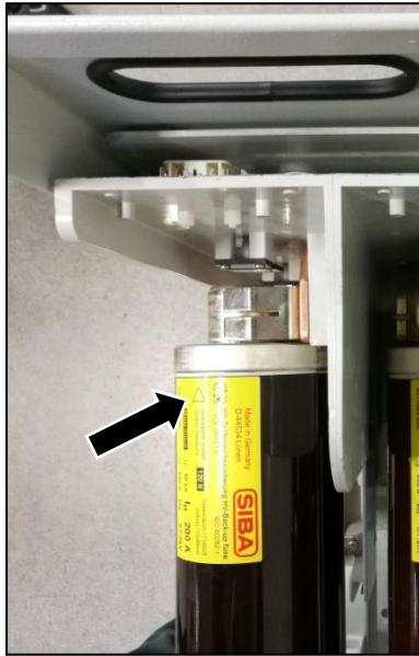
Fig. 253: HV HRC fuse-link inserted and fuse-link bracket closed in the striker area
