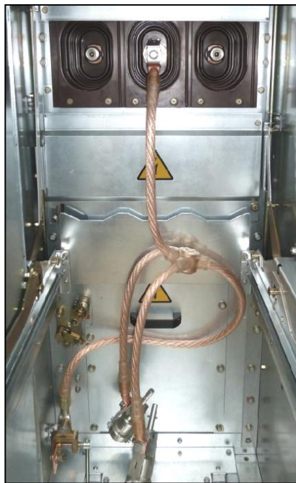
Fig. 684: Earthing tulip fixed on central bushing contact
