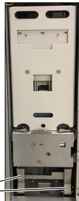
Fig. 234: Contactor panel with high-voltage door open
