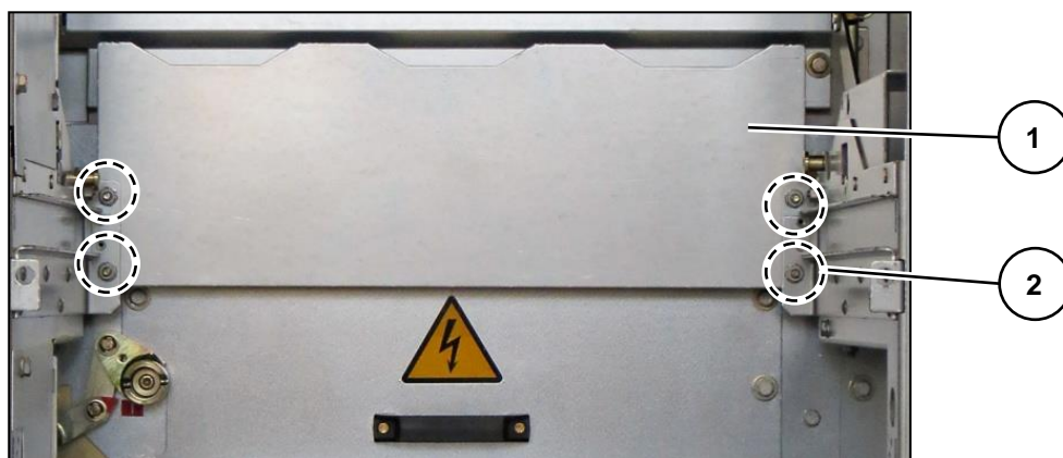
Fig. 603: 4 bolted joints on protection plate
