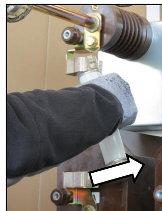
Fig. 372: Pulling off the fuse-link
