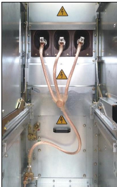
Fig. 686: Earthing device to be removed
