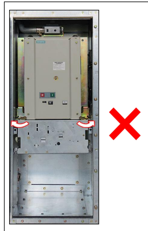
Fig. 114: Circuit-breaker panel without service truck
