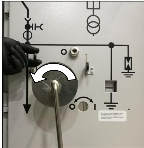
Fig. 209: Turning the racking crank counter-clockwise
