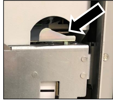
Fig. 243: Contactor truck locked
