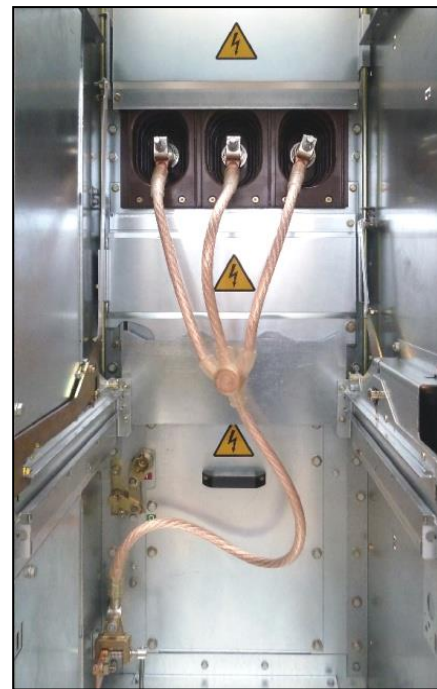
Fig. 685: Earthing device completely mounted
