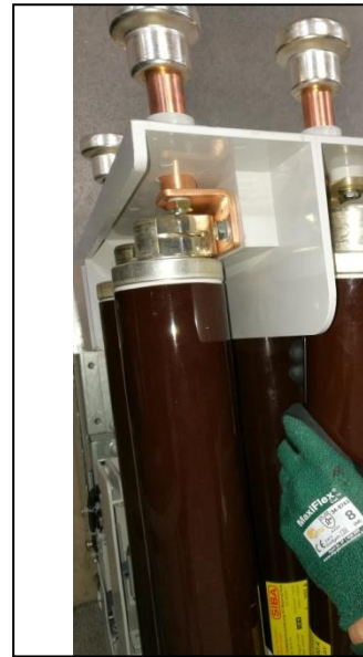
Fig. 254: HV HRC fuse-link inserted and fuse-link bracket closed on the opposite side of striker area
