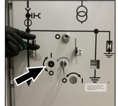
Fig. 187: Operating shaft for racking crank
