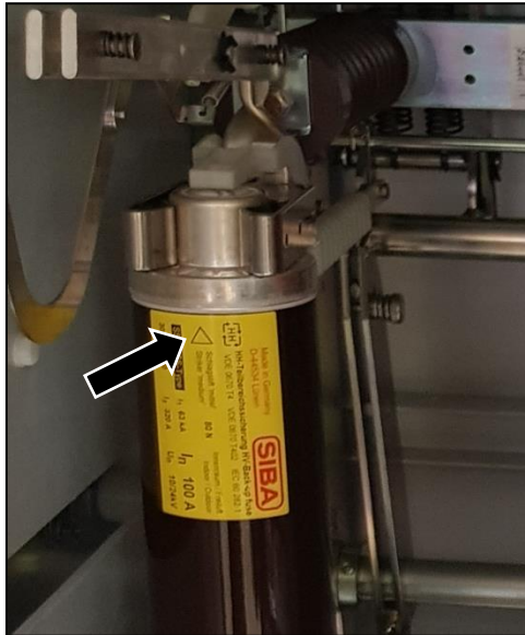
Fig. 423: The position of the striker
