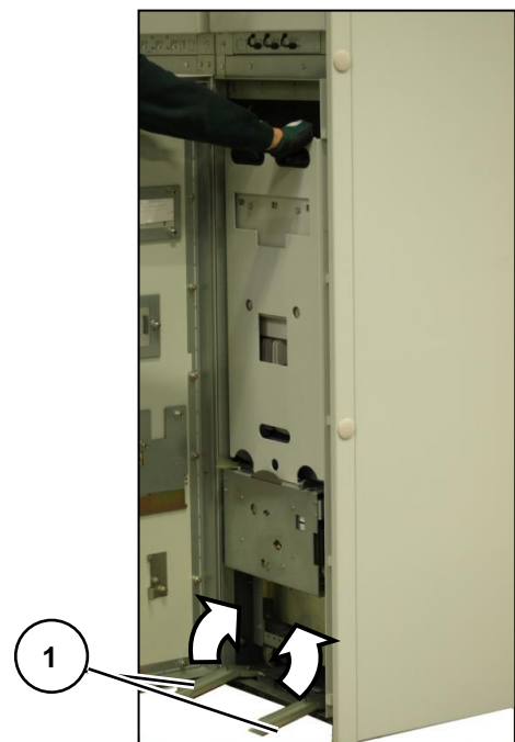
Fig. 241: Lifting the ramps
