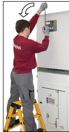
Fig. 519: Opening the busbar earthing switch using an electrician's ladder
