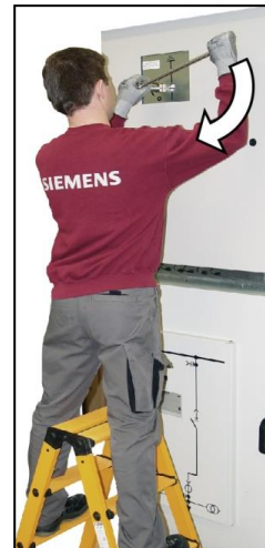
Fig. 506: Closing the busbar earthing switch using an electrician's ladder
