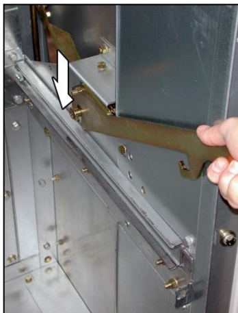
Fig. 530: Pushing on the slip-on lever
