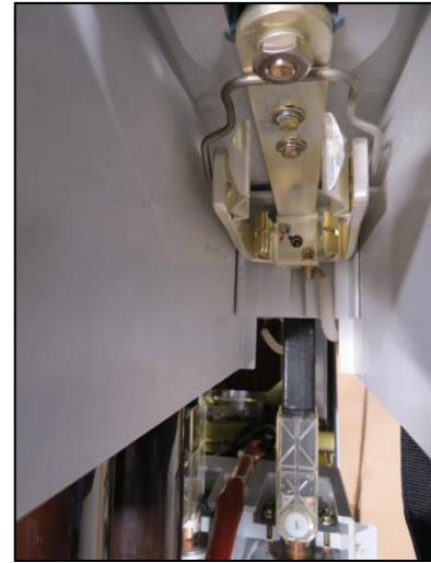
Fig. 258: HV HRC fuse-link removed on the opposite side of the striker area
