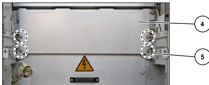
Fig. 590: 4 bolted joints on protection plate of switching-device compartment
