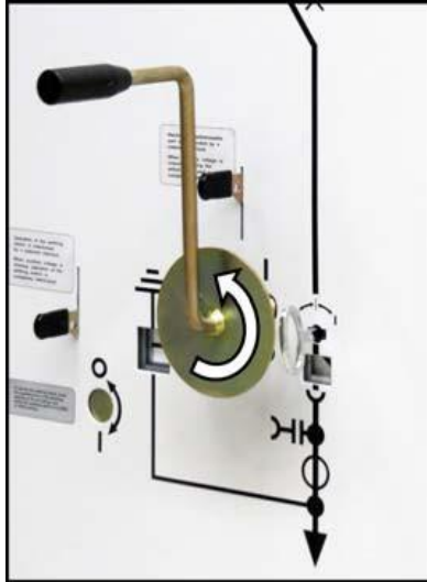
Fig. 72: Turning the racking crank counter-clockwise
