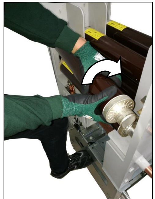
Fig. 252: Inserting the HV HRC fuse-link on the opposite side of the striker area
