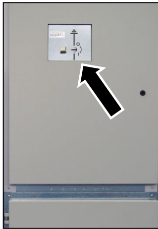
Fig. 510: Control elements of earthing switch for busbar system
