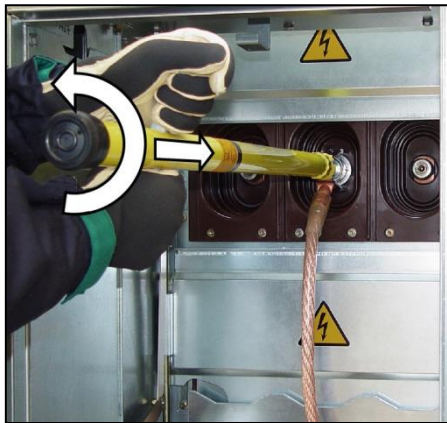
Fig. 689: Detaching the earthing tulip
