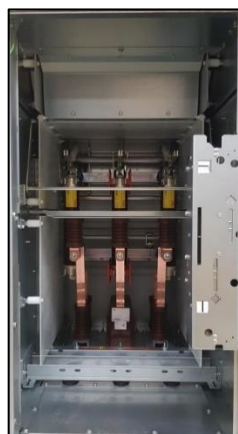
Fig. 554: Switch-disconnector panel only: Switching-device / connection compartment accessible
