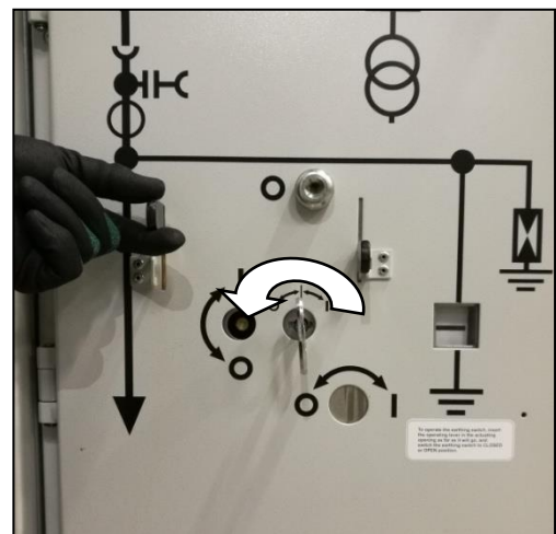
Fig. 196: Turning the double-bit key counter-clockwise
