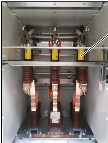
Fig. 418: Front view: Arrangement of HV HRC fuse-links (high-voltage door open )
