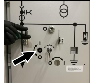
Fig. 194: Operating shaft for racking crank
