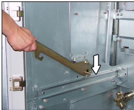
Fig. 525: Pushing on the slip-on lever
