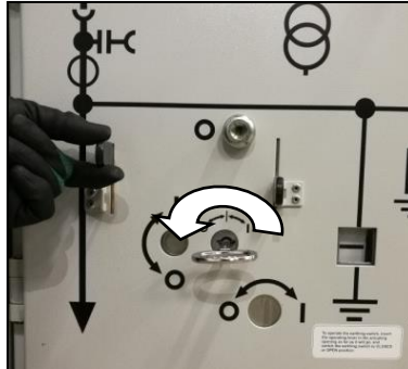
Fig. 193: Turning the double-bit key counter-clockwise
