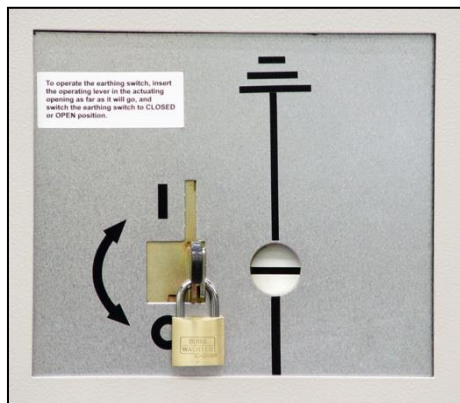
Fig. 522: Operating slide on busbar earthing switch padlocked
