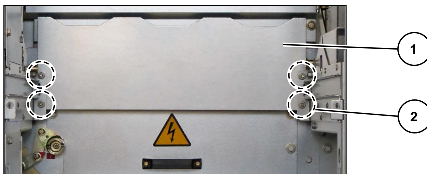
Fig. 586: 4 bolted joints on protection plate
