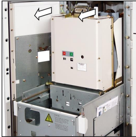
Fig. 119: Pulling out the withdrawable circuit-breaker type 3AE1
