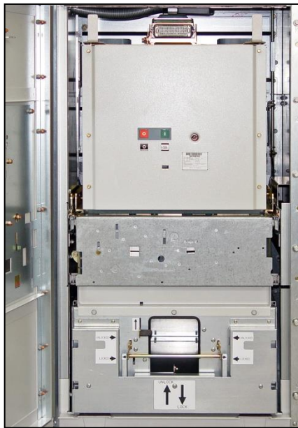
Fig. 144: Circuit-breaker panel with high-voltage door open
