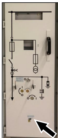
Fig. 201: Manual unlocking, padlocked
