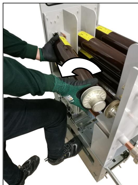
Fig. 248: Opening the fuse-link bracket on the opposite side of the striker area (contact tulip side of contactor truck)
