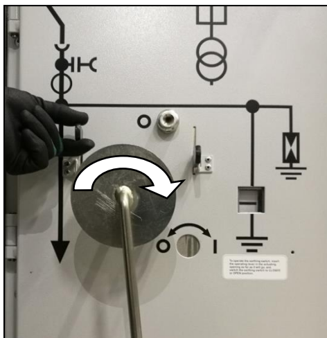
Fig. 188: Turning the racking crank clockwise
