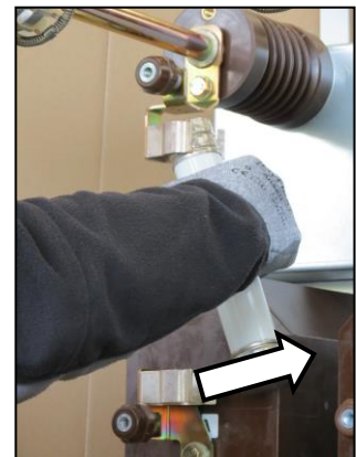
Fig. 175: Pulling off the fuse-link
