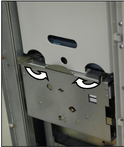
Fig. 242: Interlocking the contactor truck
