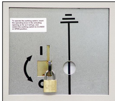
Fig. 509: Operating slide on busbar earthing switch padlocked
