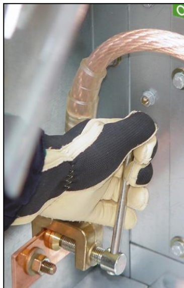
Fig. 677: Bolting earthing clamp
