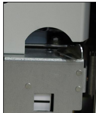
Fig. 228: Contactor truck unlocked
