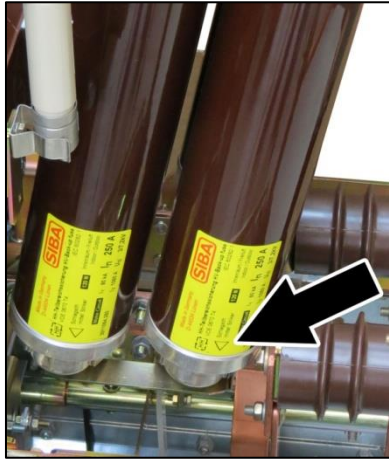
Fig. 351: Striker pin pointing to lower clamp
