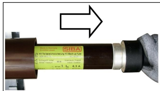
Fig. 472: Pulling fuse-link out of the housing
