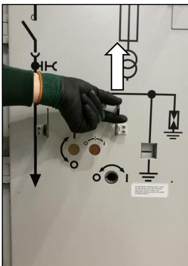
Fig. 213: Lifting the operating slide
