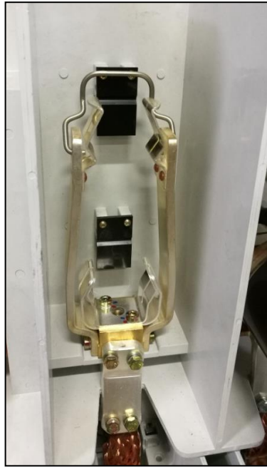
Fig. 257: HV HRC fuse-link removed in the striker area
