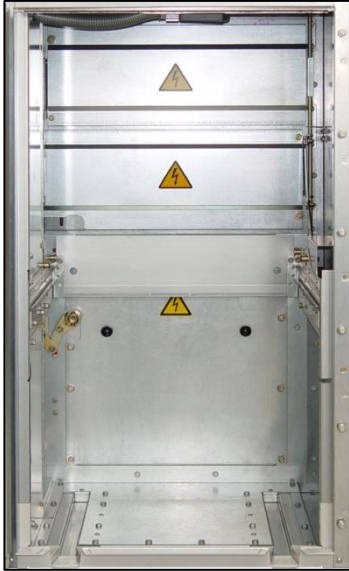
Fig. 155: Panel prepared to insert circuit-breaker truck
