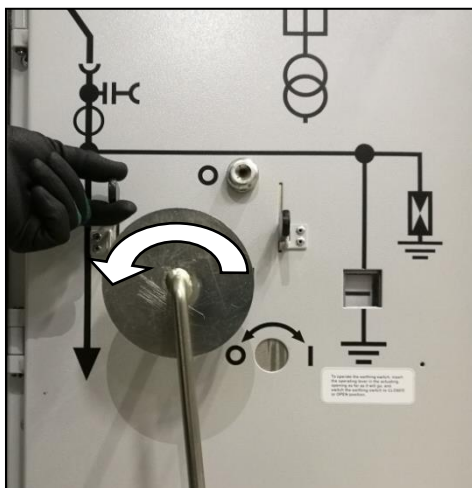
Fig. 195: Turning the racking crank counter-clockwise
