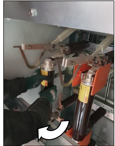
Fig. 420: Removing the fuse-link on the opposite side of striker area (bottom side)
