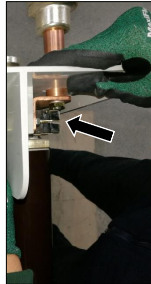
Fig. 250: HV HRC fuse-link removed on the opposite side of the striker area
