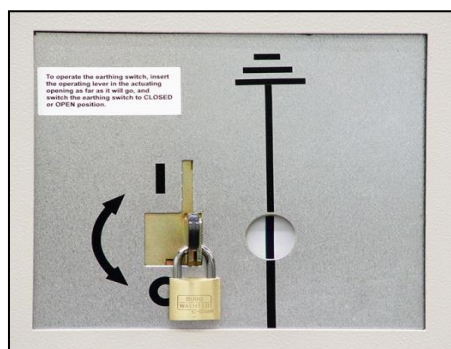
Fig. 513: Operating slide on busbar earthing switch padlocked
