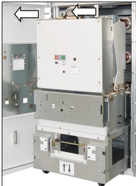
Fig. 148: Pulling out the circuit-breaker truck
