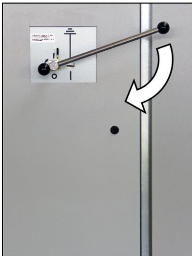
Fig. 505: Closing the busbar earthing switch
