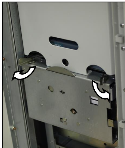
Fig. 227: Releasing the interlocking with the panel
