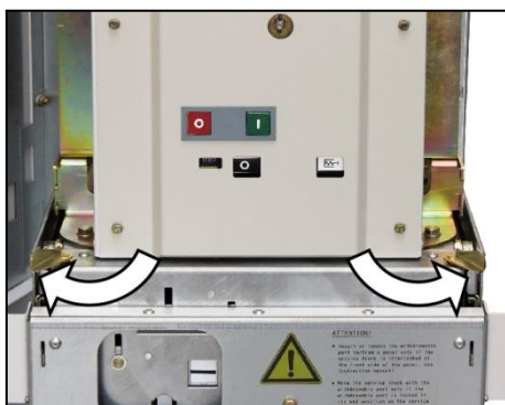
Fig. 134: Releasing the interlocking of the withdrawable circuit-breaker
