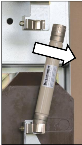
Fig. 368: Pulling off the fuse-link
