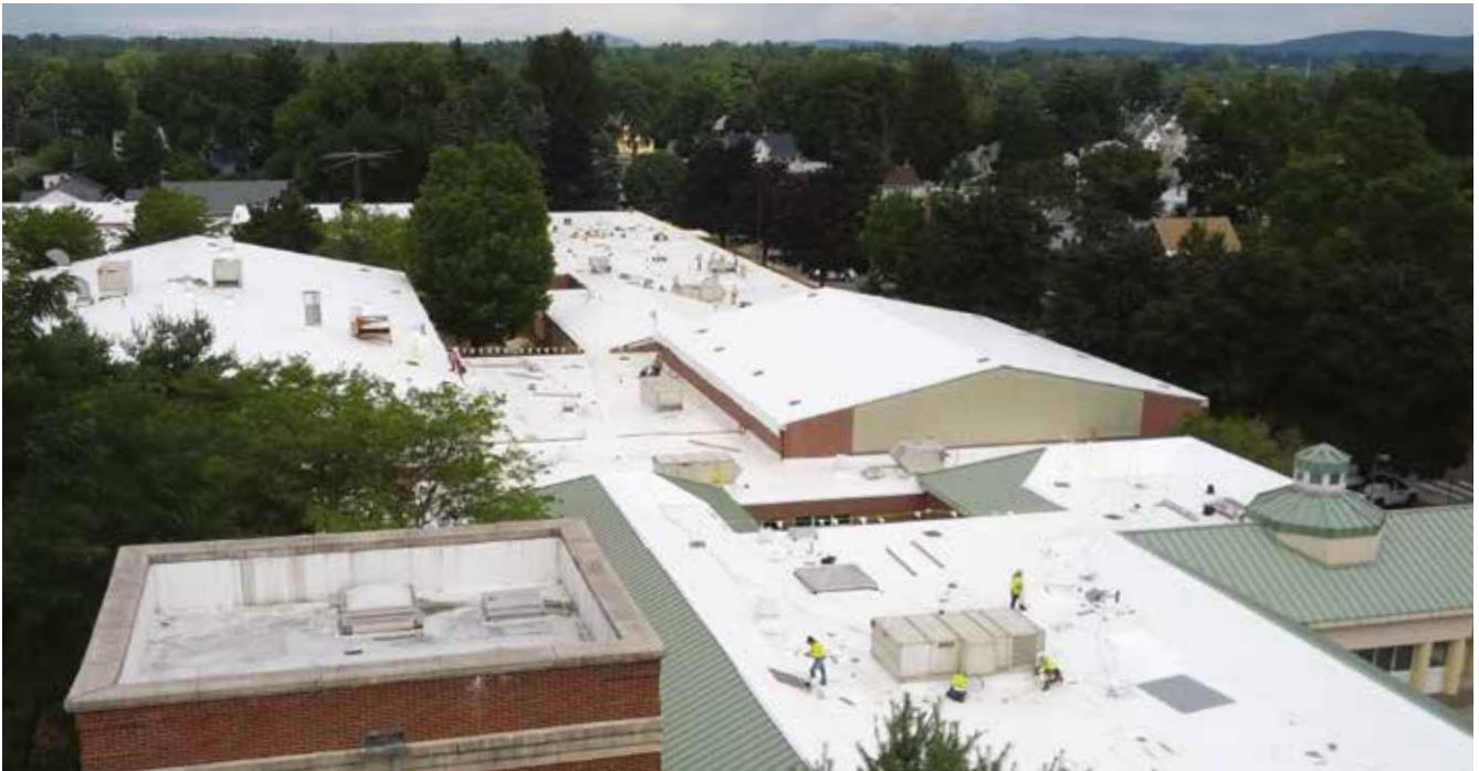
Renovations at Westfield Technical Academy
