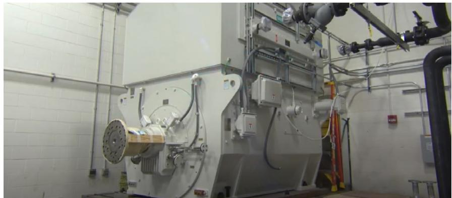
A 5 megawatt motor newly installed in the Notre Dame Turbomachinery Lab drive train compartment is waiting to couple to its first test equipment.
