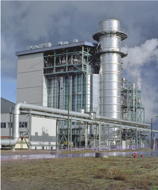
The automation solution from Siemens integrates 16 plant clusters with different network infrastructures.
