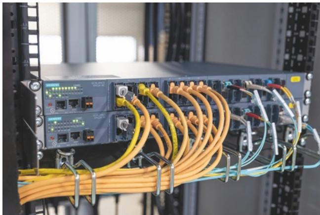
Heart of the new production network: Two of the altogether 32 SCALANCE XR524 switches, which enable the communication over a redundant Industrial Ethernet ring at up to 1 Gigabit.
