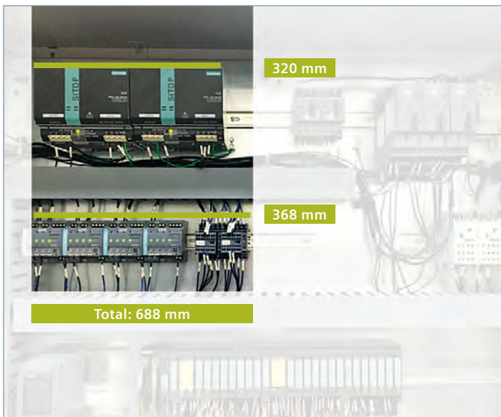
Figure 2. The Siemens SITOP PSU8600 power supply system requires half the cabinet space than the previous SITOP solution it replaced. At left is previous cabinet configuration using two SITOP 24 V / 20 A modules and four PSE200U for circuit protection, with significant wiring required. At right is the upgraded configuration: One Siemens SITOP PSU8600 5-28 V / 40 A basic module and three SITOP CNX8600 expansion modules for power, integrated circuit protection, and diagnostics via PROFINET.
